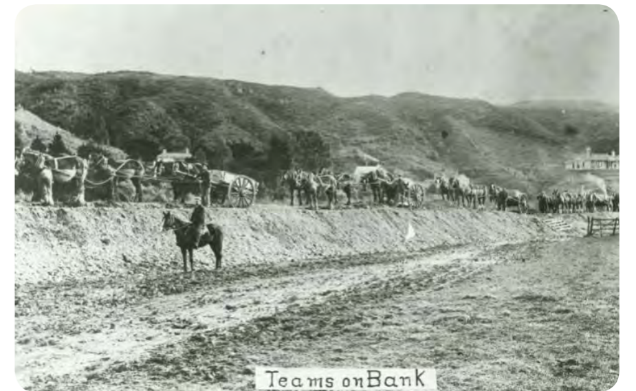
FIGURE 4 1902 Stopbank construction
