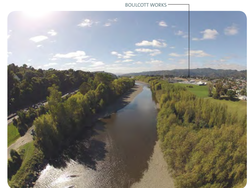
FIGURE 9 Boulcott area works
